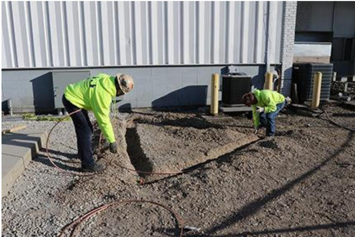
GROUNDING — Nick Bunch (left) and Kent Glassburn (right) from J&J electric work on a grounding grid at Kokomo Auto World.
